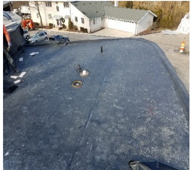
Rubber roof on the east vestibule
